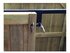
**Step 6:** Now close both doors and hold in place by latches. If the surface is flat, the top of both doors should be aligned and will have a 10-15mm gap between them (as shown below) to avoid rubbing against each other while opening and closing. If door tops are not aligned, use suitable packers e.g. washers etc. as required under a corner of the store to align them.
