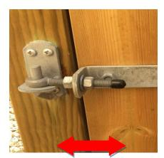
Shutting Gaps Adjustment by winding Nuts in or out as required
