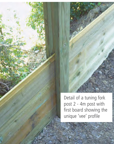
Close up of the interlocking vee section
