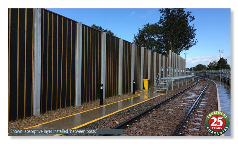
The Jakoustic® Commercial & Highway Absorptive barrier system has been designed for commercial and highway applications, providing the same level of noise protection as the original Jakoustic® Absorptive barrier, but it can be additionally UKCA marked as a whole system for road infrastructure.
