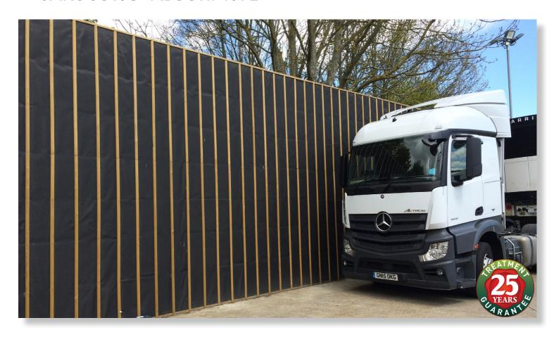
The Jakoustic® Absorptive barrier is designed specifically to keep noise within a contained space and is typically used around continuous power supply generators, air conditioner compressors, waste compactors and goods loading areas.
