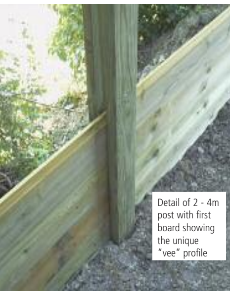
Close up of the interlocking vee section
