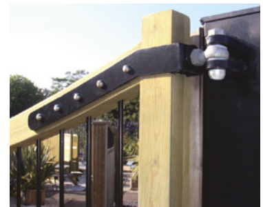
Hinge detail of Cathedral Gate
