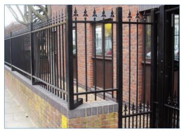
Ornamental fencing fitted with cranked posts mounted on existing wall with special width full height panel installed adjacent to the pedestrian gate
