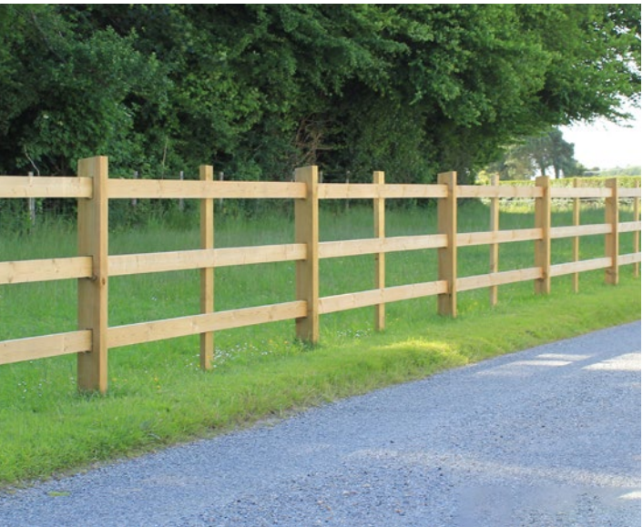
Image showing intermediate post in Post & Rail Morticed system
