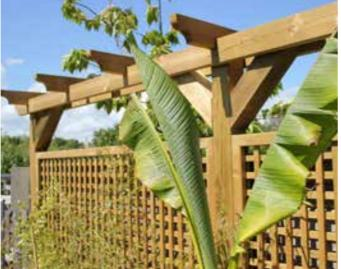
75mm nails (800210 - 1kg) are used for the majority of the construction, but you should use 100mm nails (800310 - 1kg) for the in-line braces. When using nails to join two timber parts we recommend drilling a pilot hole through the first part to insert the nail through, this enables the nail to be driven easily into the other part of the structure, and reduces the likelihood of splitting.
