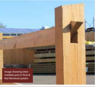
Allow one post and one prick post for every 2.85m of fence, plus one post for the end of the run. Allow three rails per 2.85m run of 3-rail fence, and four rails per 2.85m of 4-rail fence.
