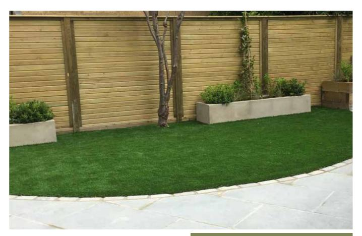
Panels are 1.83m wide, with heights of 0.91m to 1.83m. Supporting rails are 45mm x 51mm and sides are 70mm x 51mm. Panels are available in five heights from 0.91m to 1.83m x 1.83mm wide with the option to use a panel width cut-down kit if required. Horizontal Tongue and Groove Effect panels have 21 pales.
