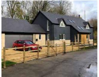
Allow one post for every 1.85m of fence, plus one for the end of the run.
