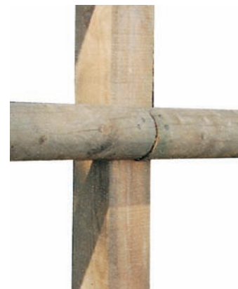
Detail of rail to post fixing
