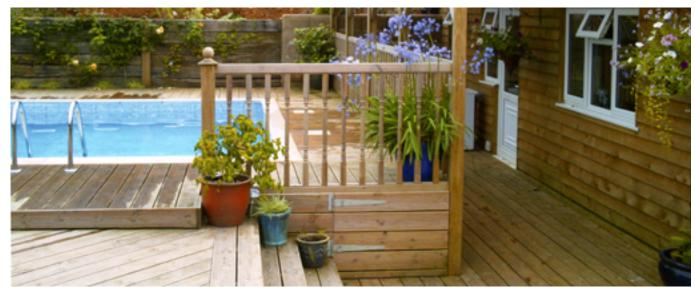
Decks are constructed with spaces between boards to aid drainage and to allow for the natural expansion and shrinkage of the timber, while all fixings and fastenings are non-rusting to ensure an extra-long life.
