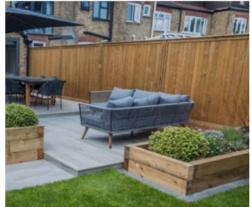
The centre of the panel is given additional support with one 70mm wide rail for heights up to 1.22m, and two rails for heights of 1.52m and above. Panels are 1.83m wide, available in five heights from 0.91m to 1.83m with the option to use a panel width cutdown kit if required. Top and bottom rails are 70mm x 51mm planed with sides of 45mm x 51mm. Standard Tongue and Groove Effect panels have 21 pales.
