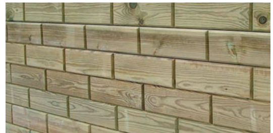
Wall/fence made from 140mm grooved face Jakwall
