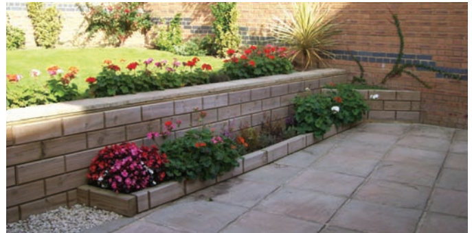
Retaining wall and Raised beds created using 140mm grooved face Jakwall
